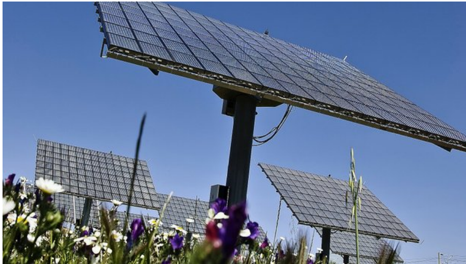
Concentrix panels sit on steel poles and turn to follow the sun across the sky. And they use lenses to focus the sun's rays on highly efficient photovoltaic chips like those use on spacecraft. — Concentrix Solar
