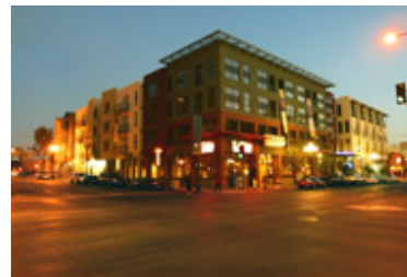
OliverMcMillan is the largest private landowner in downtown San Diego. Pictured is its mixed-use Lofts at 777 Sixth project.
